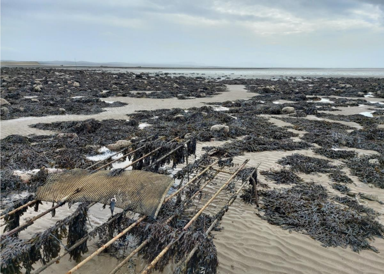
Figure A4.5 View of Abandoned Trestles with Active Aquaculture Sites in the Background
